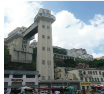
Vertical pedestrian mover in Brazil
