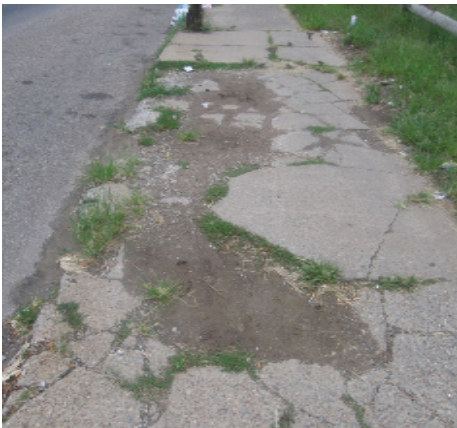
Sidewalk on Forbes Avenue, Uptown
